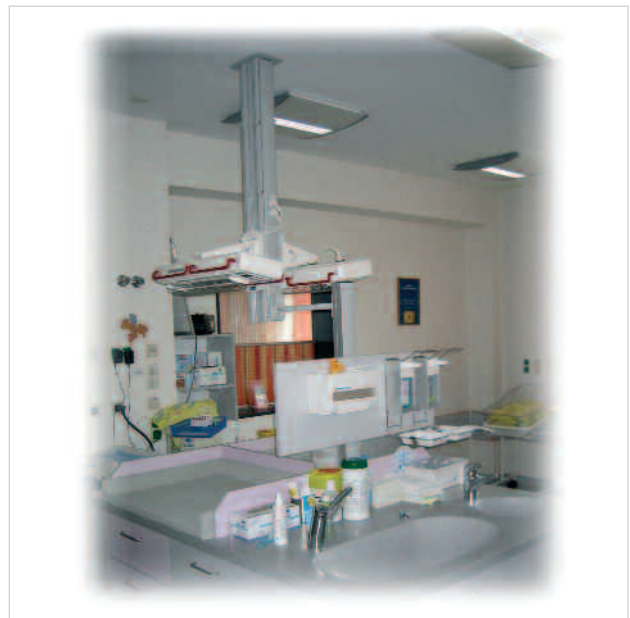
Application (ceiling assembly) on a diaper-changing unit for newborns
