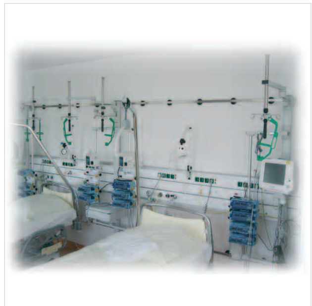
Fixing to wall supply duct and standard runner on the intensive-care station
